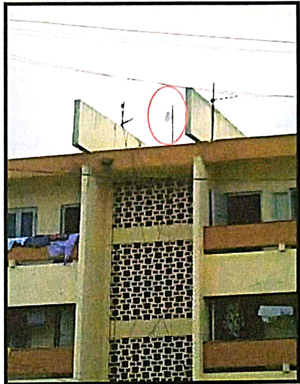
Wi-Fi Antena on UGC Staff Quarter (Signal Receiver)
